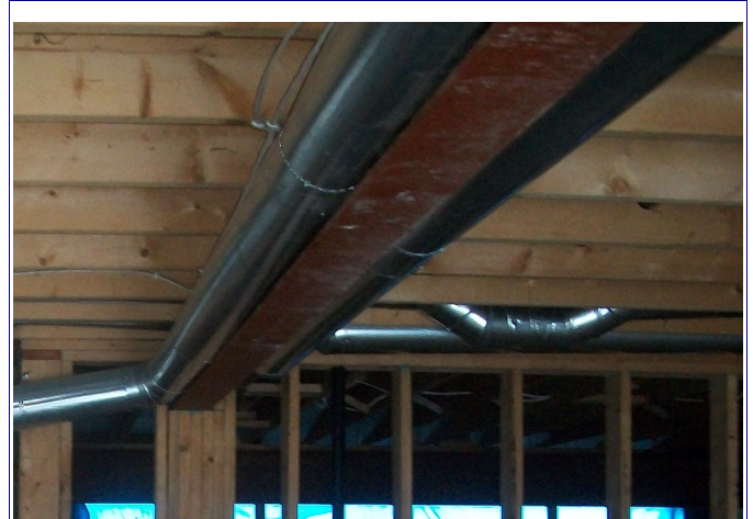
Illustration 4.: Wood Joists and Steel Beam
