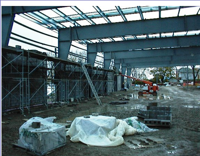
Illustration 3.: Rigid Frame Steel Structure
