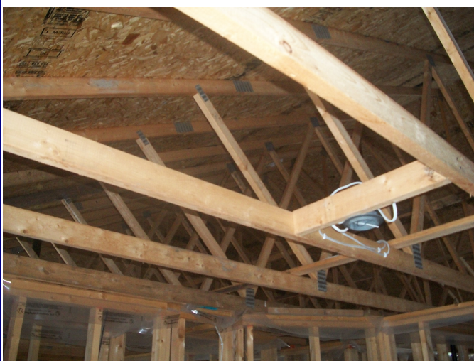
Illustration 1.: Wood Trusses
