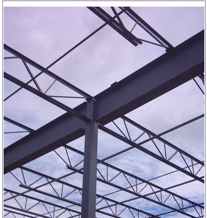
Illustration 2.: Open Web Steel Joists
